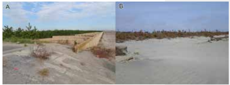
Figure 12: Damage conditions of sand embankments and preserved forests: (A) photograph taken on November 11, 2010 by Dr. Kentaro Imai, Tohoku University), and (B) photograph taken on May 5, 2011 (Sugawara and Minoura, 2013).
