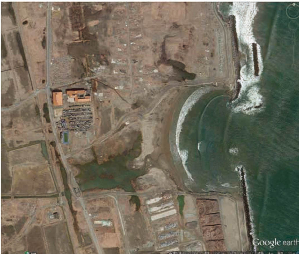
Figure 10: Overview of old Nakahama Elementary School of Yamamoto town (building with orange roof in left center side) and “Tsunami Bay (eroded arc-shaped coast in right center side).”
