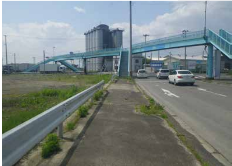
Figure 16: Pedestrian bridge at the cross junction of the prefectural road no. 10 and the city road.
